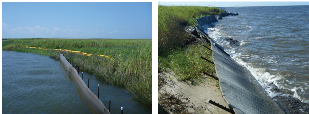
Figure 3-3. Shoreline barriers used during the Deepwater Horizon oil spill. Filter fences require many stakes. Usually there is not enough time to deploy this type of barrier after a spill, they have limited effectiveness, and they are difficult to remove. The hard boom has become stranded on the marsh. Photo credit: Helen Chapman (left); Thomas Minter (right).
