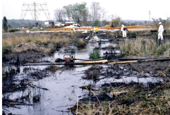
Figure 3-10. Intensive flushing operations along one of the trenches excavated at the Chalk Point, Maryland spill in April 2000. Flushing of oil from the marsh interior is very difficult. Photo credit: Jacqueline Michel.
