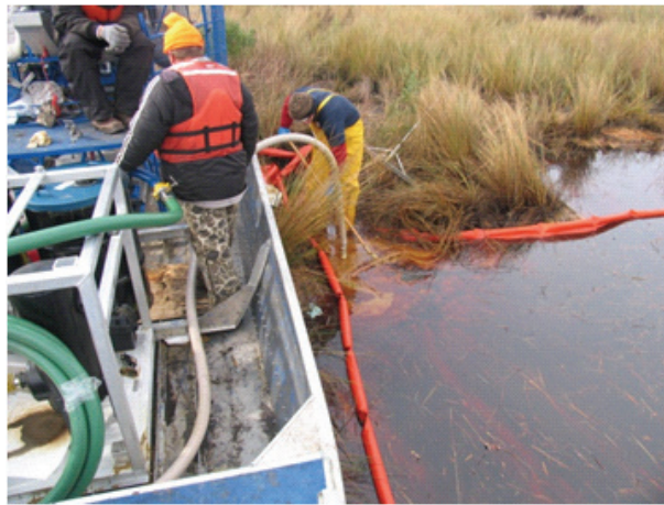
Figure 3-7. Vacuuming of thick oil from the water surface in a marsh channel, Bayou Perot, Louisiana in February 1997. Photo credit: Jacqueline Michel.
