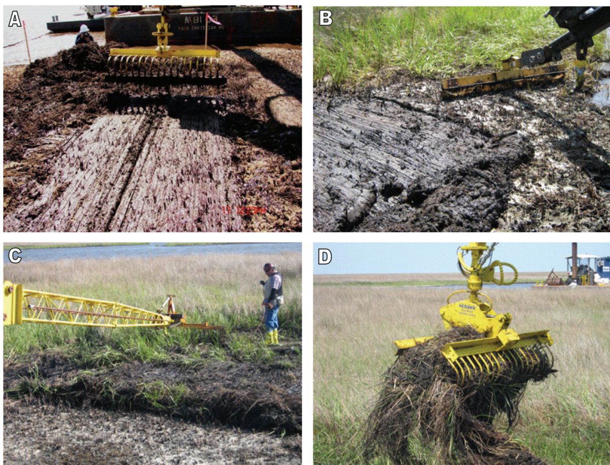
Figure 4-4. Mechanical treatment methods used to remove the thick oil and oiled vegetation mats on the marsh surface in N. Barataria Bay, Louisiana, during 2011. A: Raking of oil/mat on the outer platform would gouge the marsh soils if done too deeply. Photo credit: Jeffrey Leonick. B: Flat “squeegee” used to scrap the thick oil into piles for removal. C: Raking of the oiled wrack line had to be carefully guided to minimize removal of live vegetation. D: Grappling of the piles of oiled wrack was efficient and minimized foot traffic. Photo credit B-D: Jacqueline Michel.
